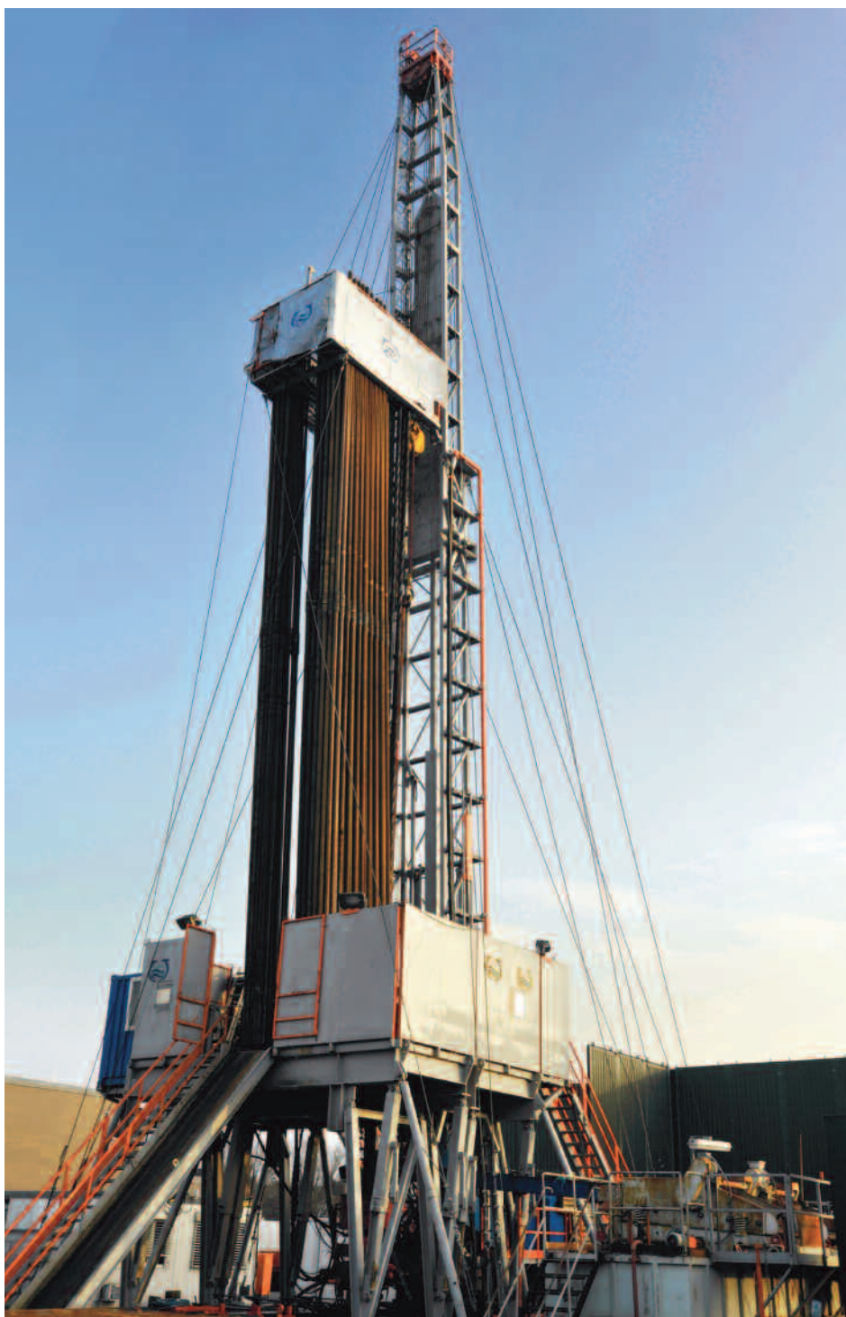
Drilling rig MR 8000
