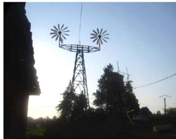
Figure 4. Wind electric pumping system at NdohDjutissa in Cameroon (Nfah and Ngundam, 2012).
