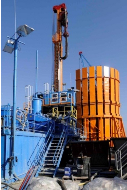
Geothermal drilling in Germany. Copyright: Kreuter
