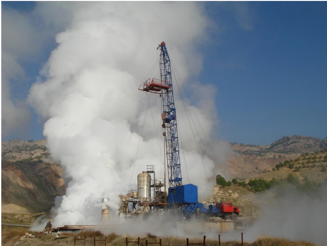
Geothermal Drilling in Turkey, Copyright: Zorlu (Turkey)
